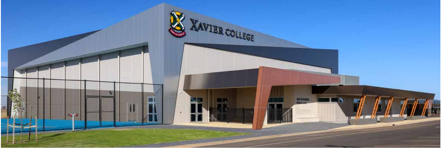
Completed gymnasium and OSHC facility at Two Wells Campus
